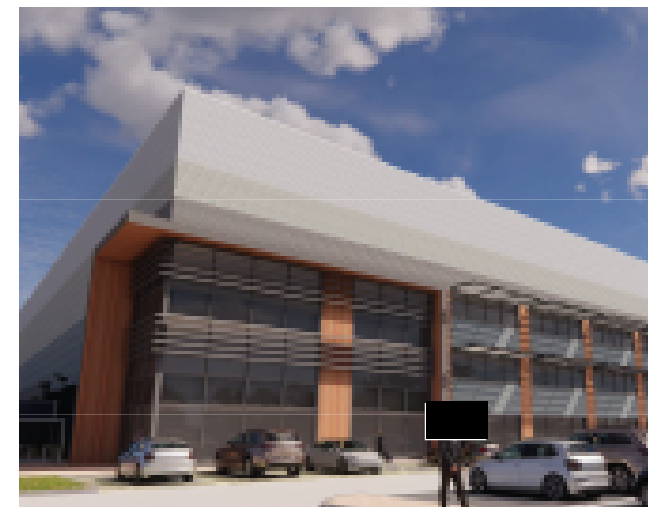
Solar shading to southern elevations
