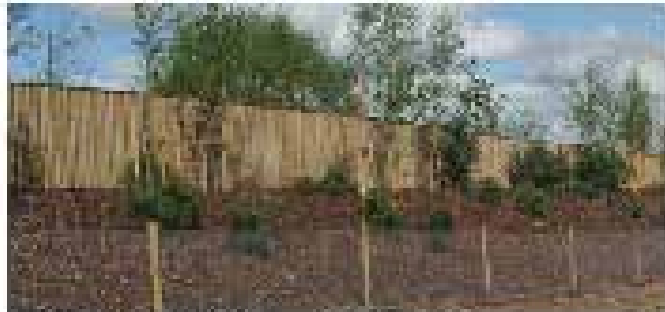
Acoustic fence in a landscaped area where vegetation is available
