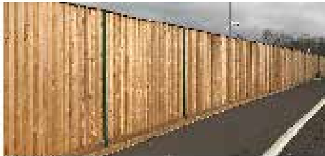
Typical Acoustic Barrier
