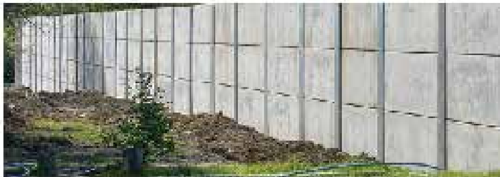
Acoustic retaining wall with vegetation, with sound-reflective from public room
