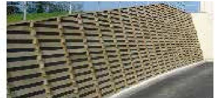
Acoustic retaining wall
